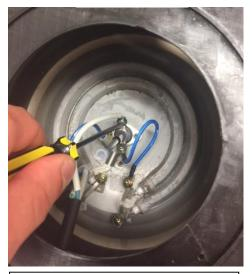
Unscrew the white wire from the thermostat. Make sure to not let the loose wire touch anything, use electric tape to tape up the loose end of the wire.
