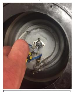
Unscrew the first screw that connects the thermostat to the boiler.
