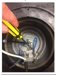
Unscrew the blue wire from the thermostat. Cover the tip of this wire the same as in step 4.
