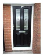
Doorways can be made much more robust, making it harder for an assailant to gain entrance. Typically, when talking about a door from a technical, security point of view, professionals will talk about points of attachment. Those are anywhere that the door is attached to the frame. Assuming that everything is locked as it should be, the more of these that the door has, the harder it is to break through the door.
