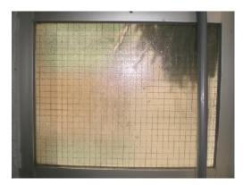
There are a number of things which can be done to a window, in order to make it stronger and better to withstand attacks. The fist of these is to replace all the window glass with the wire glass that is used in industrial facilities. While this isn't a perfect solution, it is much stronger than normal glass.
