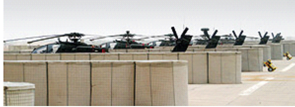
Figure 9. Helipad from HESCO Bastion 14
