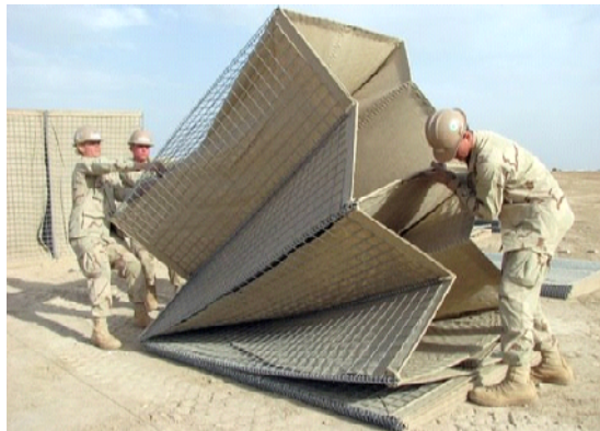
Figure 4. Deploying HESCO elements 6
