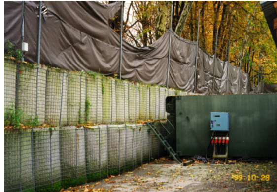
Figure 13. Fence with net against a sniper 18
