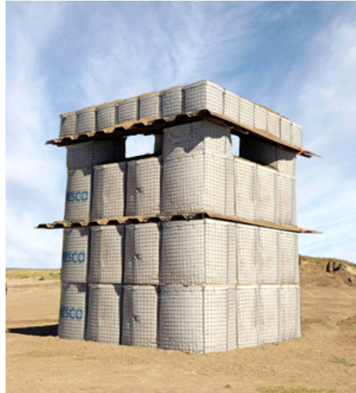
Figure 31. Elevated Observation Post 30
