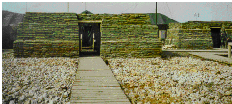
Figure 2. Personnel protective bunker 2
