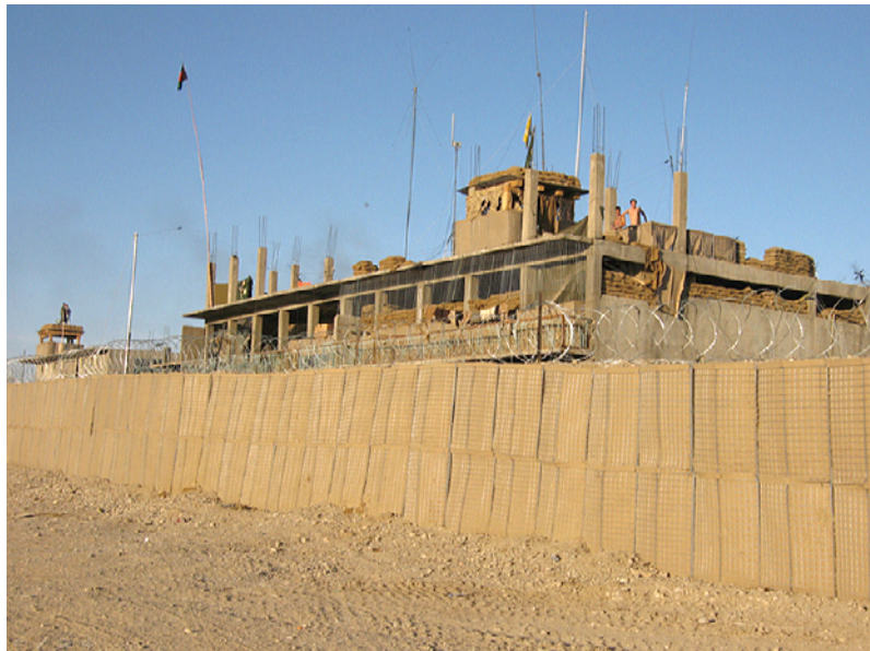
Figure 10. Defence object with HESCO wall 15
