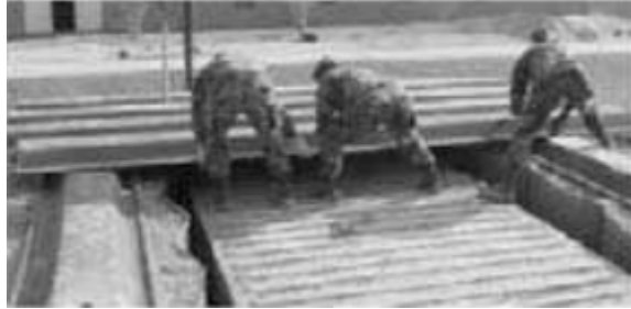
Figure 22. EOPS roof installation 25
