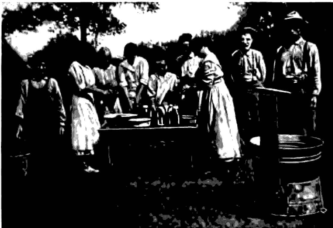
FIG. 55.—Canner made of tubs for outdoor use.
