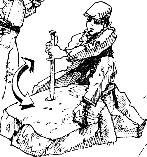
Drilling holes in a large block with a hand drill before breaking with plugs and feathers
