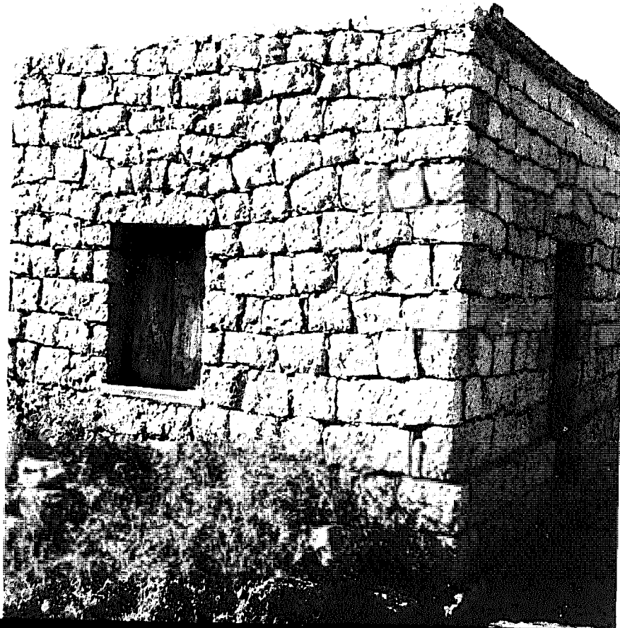
One of the greatest advantages of stone is that it can be shaped using a hammer and chisel (above). Once squared, blocks can be used to build simple buildings, such as this dry-wall dwelling, from Argentina (below).
