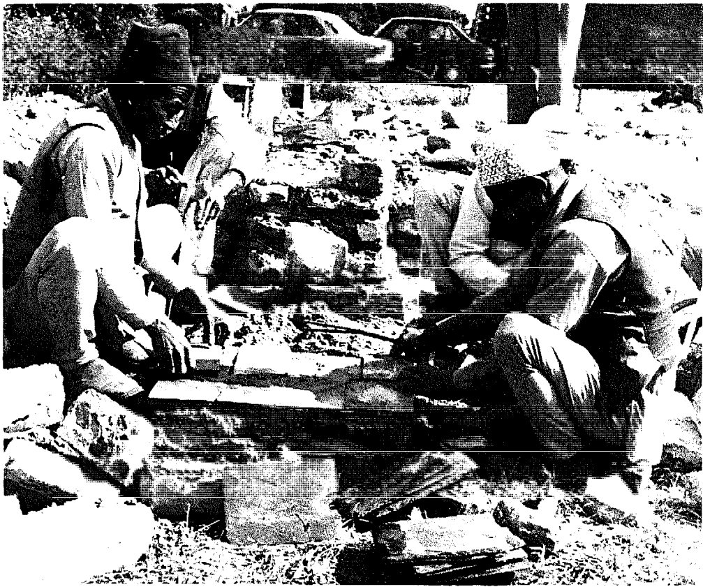
The use of slate need not be confined to roofs! Above: Laying a slate damp-proof course, Nepal. Below: Stone that was edge-bedded during construction has suffered from weathering, while the naturally bedded stone surrounding it is in far better condition.
