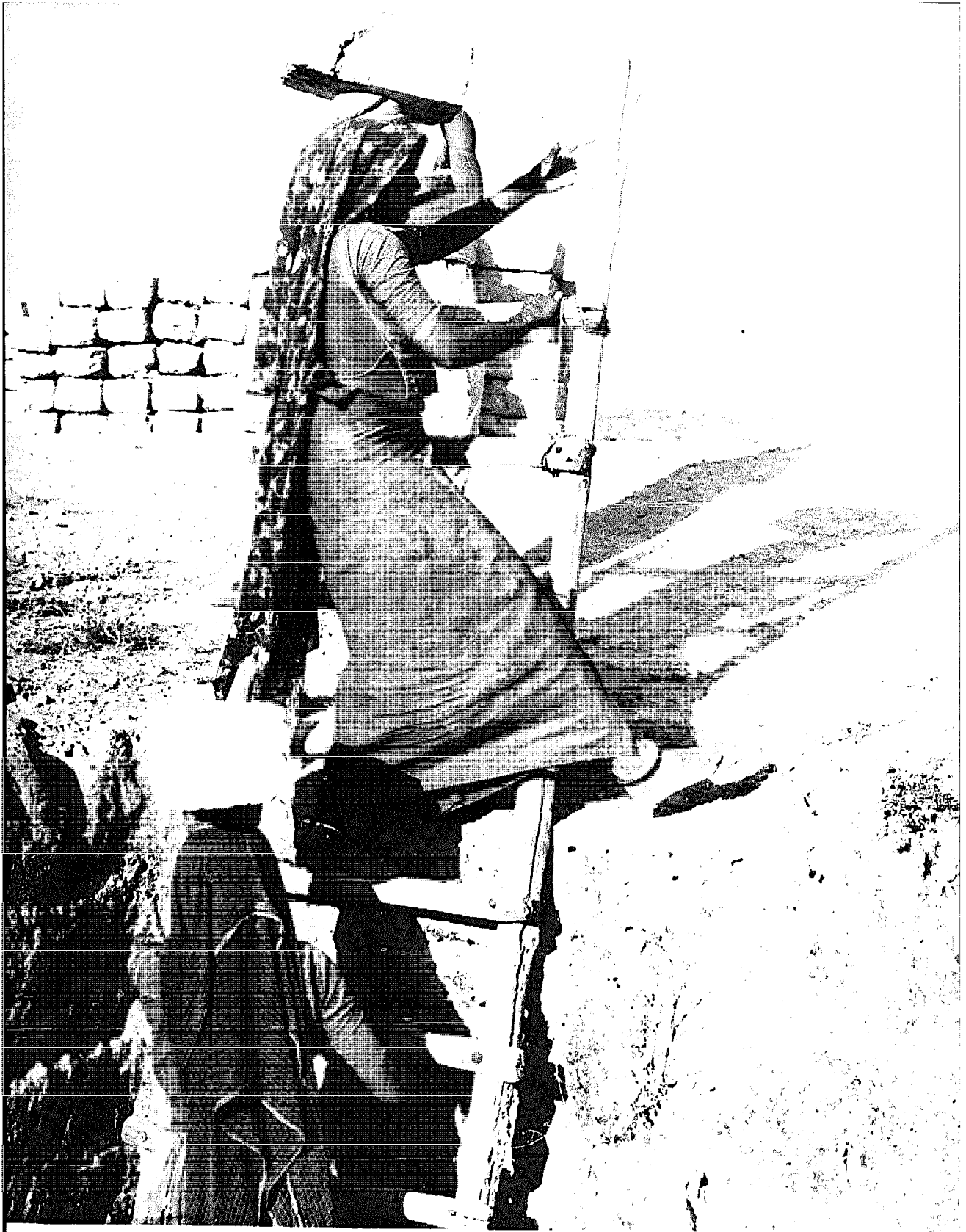
Removing building stone from an underground quarry in India.
