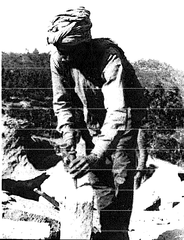
Below: Splitting sandstone, first with a hammer and chisel (left) then with a sledge-hammer peen.
