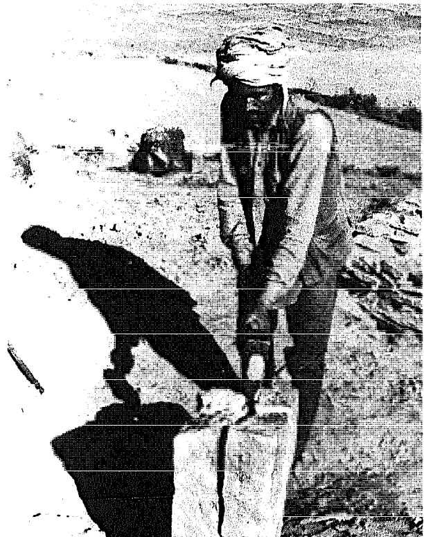
Below: Splitting sandstone, first with a hammer and chisel (left) then with a sledge-hammer peen.
