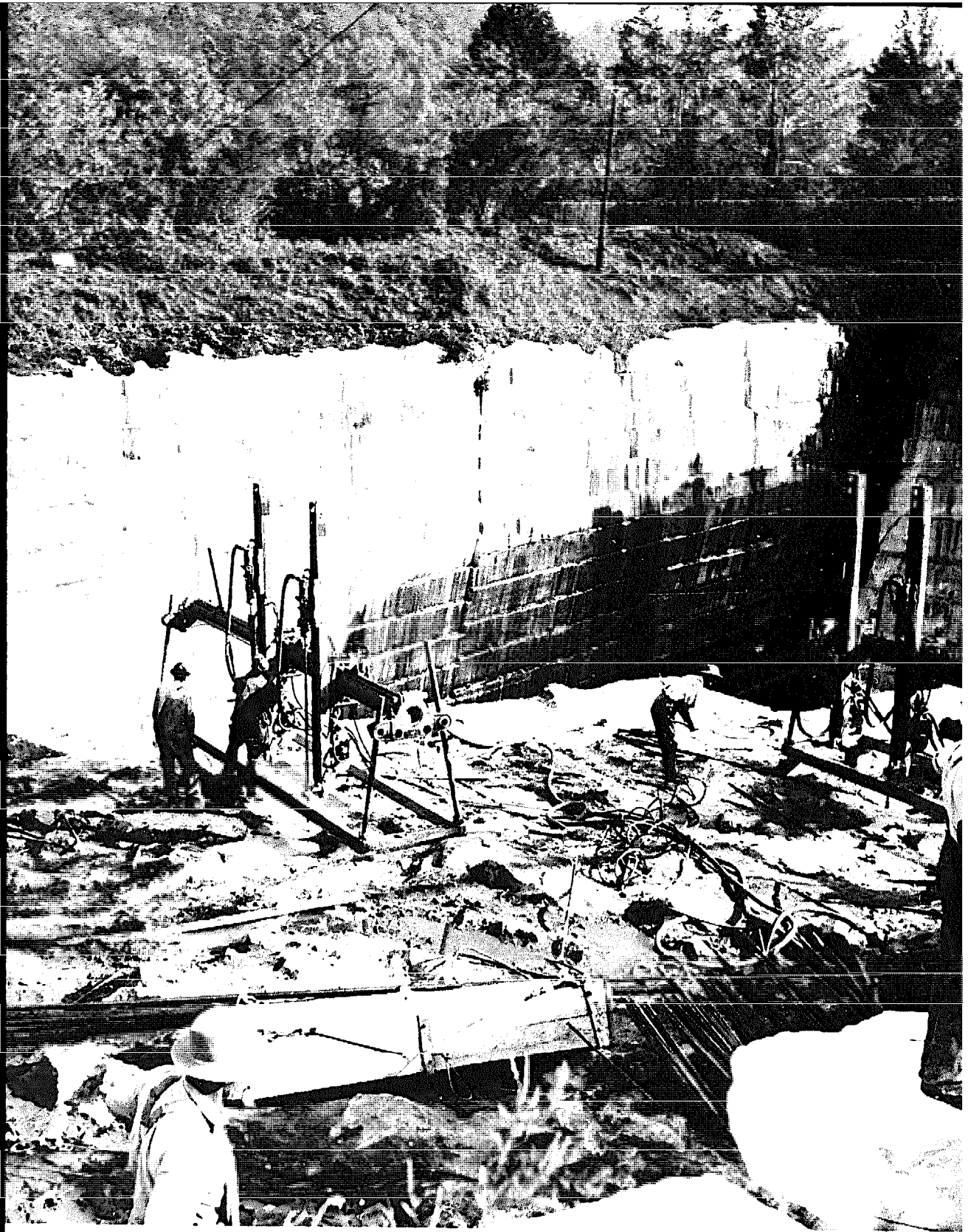
Large wagon drills are mounted on the saddles of quarry bars for accurate drilling at this marble quarry.
