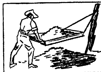
Fig. 6 - Screening the Soil
