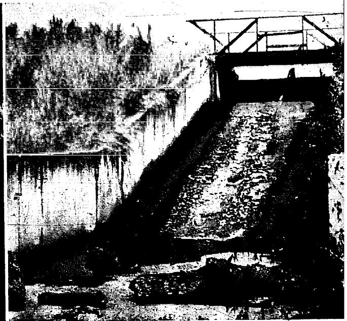
Front and back views of the concrete-lined spillway for the dam pictured at the left. Spillway is in the center of the dam and empties into the old creekbed.
