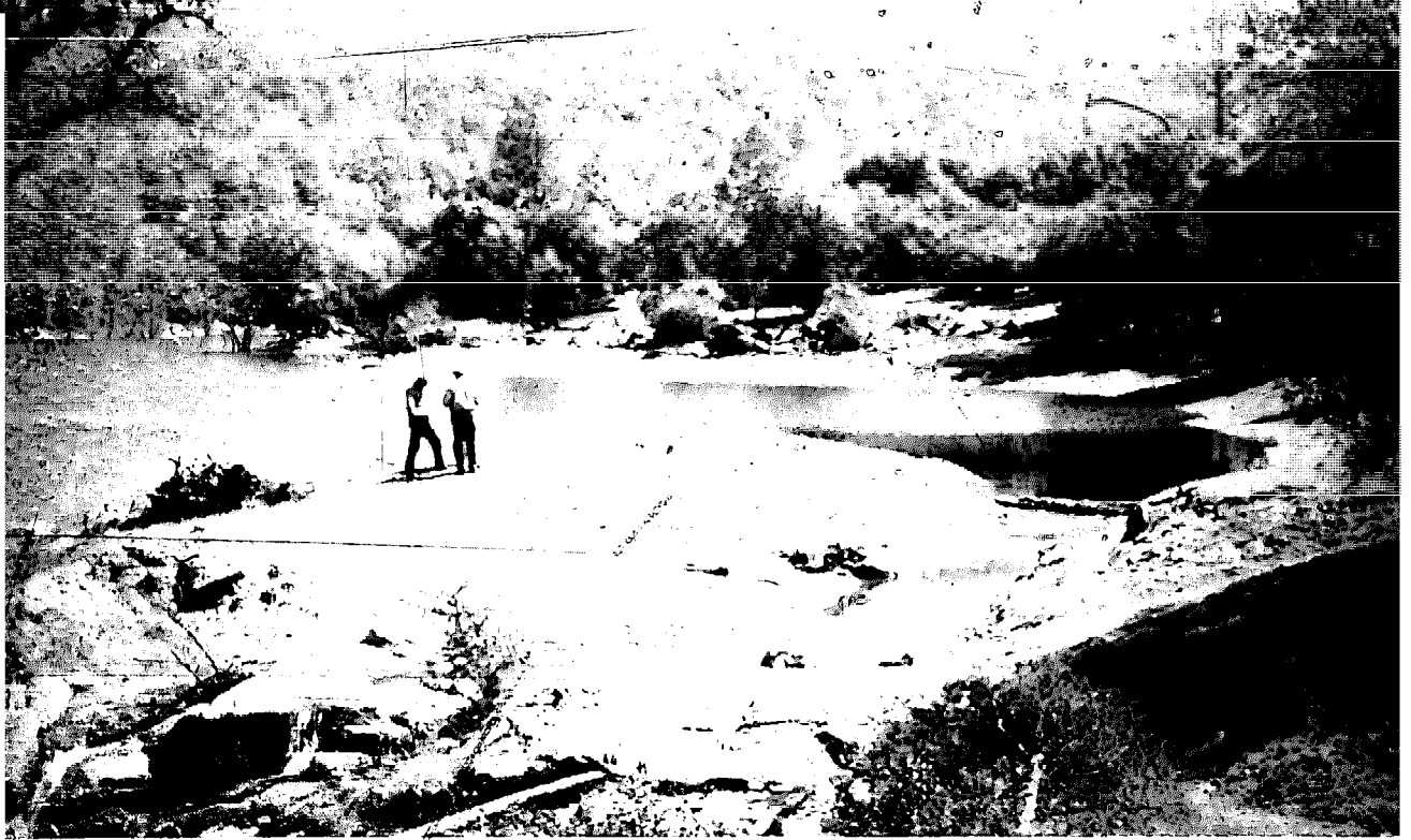
Here earth-filled sacks are used in the spillway to store additional water from late spring runoffs. Such barriers are inexpensive and easy to remove.
