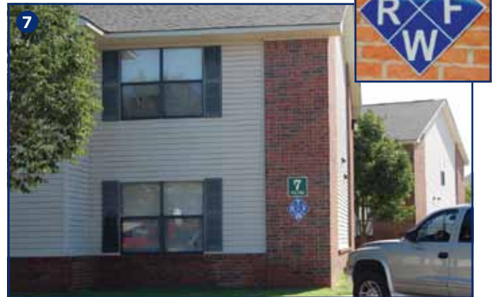
(6) The Blue Diamond Hazard Identification System placard. In this instance, it indicates the presence of truss components in the building’s roof and floors. (Photo by author.) (7) The blue diamond is located on the front corner of a lightweight wood-frame apartment building to alert firefighters. (Photo by author.)
