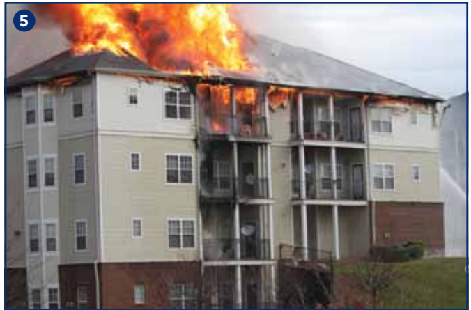
(4) Polyurethane foam adhesive was used to attach gypsum ceiling board to the wooden structural frame in the void space between floors. The floor voids are typically 14 feet x 48 feet x 20 inches per modular unit, which equals approximately 1,300 cubic feet, and may have multiple attached units. It is doubtful that the code developers thought beyond the 1,000-square-foot requirement using the length x width standard when developing the trigger for draftstopping of concealed spaces. Also, note the small dimension finger-jointed truss and the exposed back side of the foam board wall insulation. This void space creates a very effective “fire box.” [Photo courtesy of the Acushnet (MA) Fire Department.] (5) Fire entering the void space can become a structure fire on steroids, especially if it becomes wind driven. This fire started on the exterior of the structure and rapidly spread up the vinyl siding, breaching the vinyl soffit, and quickly involved the attic voids. The building’s sprinklers did not activate because of the fire’s location. [Photo courtesy of the Sterling (VA) Volunteer Fire Company.]
