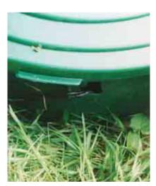
Just below the rim of the rain butt we drill a hole. Through this can run all the electric cables to the submersion pump and the circulation pump, without the lid of the rain butt having to be removed.
