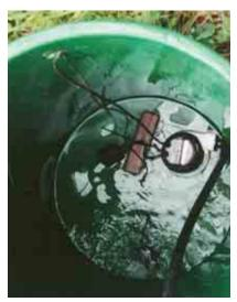
Here we can see the submersion pump sitting in the rain butt. The sensor normally floats up and down with the level of the water. I have fixed the sensor a little below this with a brick. In this way the submersion pump can continue to pump for a little longer before it cuts out.
